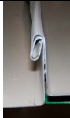
Finished QuadLok Seam
