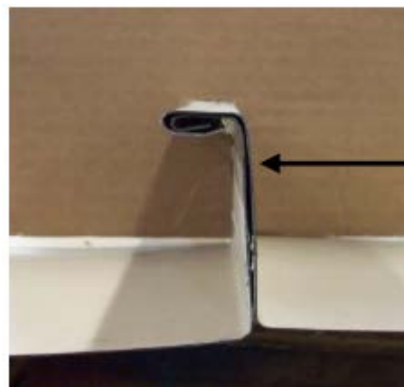
Finished TripleLok Seam Profile
