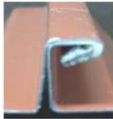
Finished TripleLok Seam Profile
